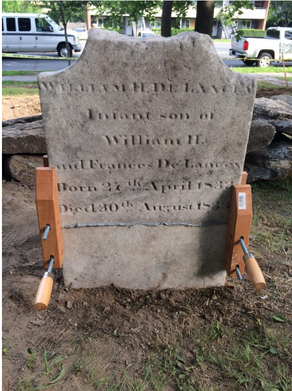
The headstone of William H. DeLancey, which was found on the ground broken into two pieces and dislocated from its place within the site, was cleaned of soil and bio-growth, and reset after reattaching with structural adhesives.
